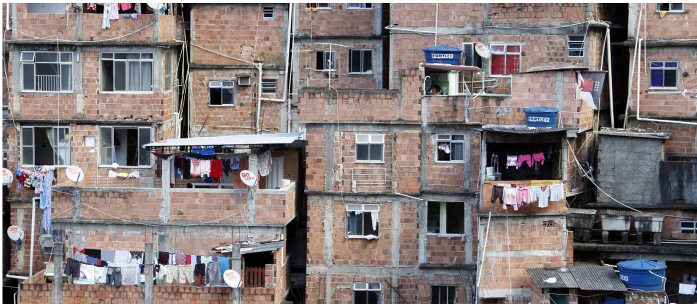
Figure 23 Typical informal occupation in Brazilian favelas. The buildings are based on a simple constructive system of pillars, beams and concrete slabs. Source: www.oglobo.globo.com
